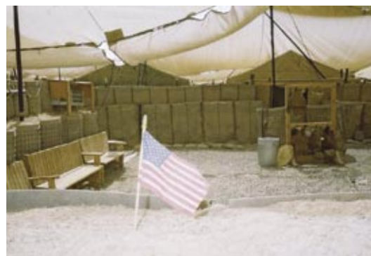
Areas of the Camp Taqaddum in central Iraq were surrounded by HESCO barriers—large containers filled with sand to protect patients and staff from insurgent attacks.
