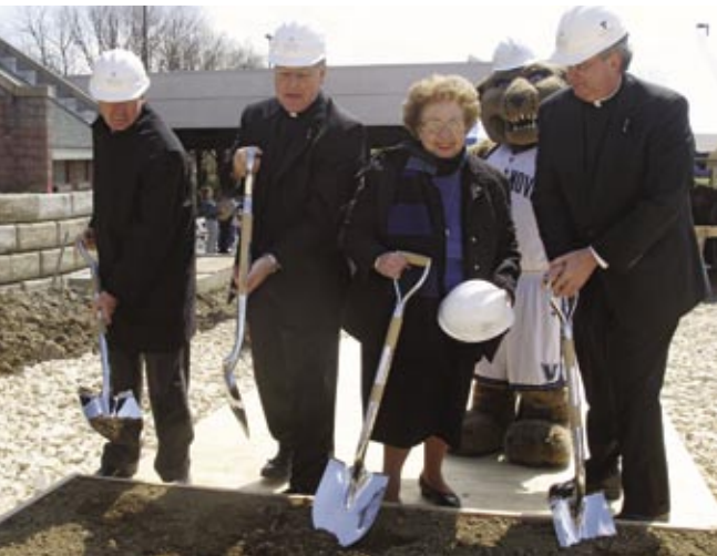
Cheered on by the Wildcat sporting a hard hat, these Villanovans participated in the April 10 groundbreaking for the new Nursing facility. They are (from left) John G. Drosdick '65 Ch.E., chairman of Villanova's Board of Trustees; the Very Rev. Donald F. Reilly, O.S.A., '71 A&S, D. Min., Prior Provincial of the Province of St. Thomas of Villanova; Dr. M. Louise Fitzpatrick, Connelly Endowed Dean and Professor; and the Rev. Peter M. Donohue, O.S.A., '75 A&S, University president.
